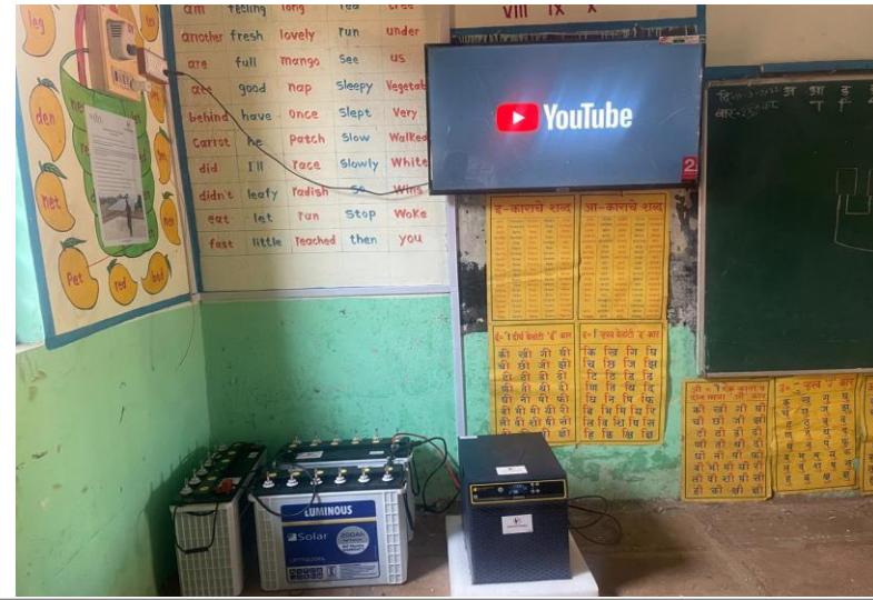
Solar Panels installed over roof
