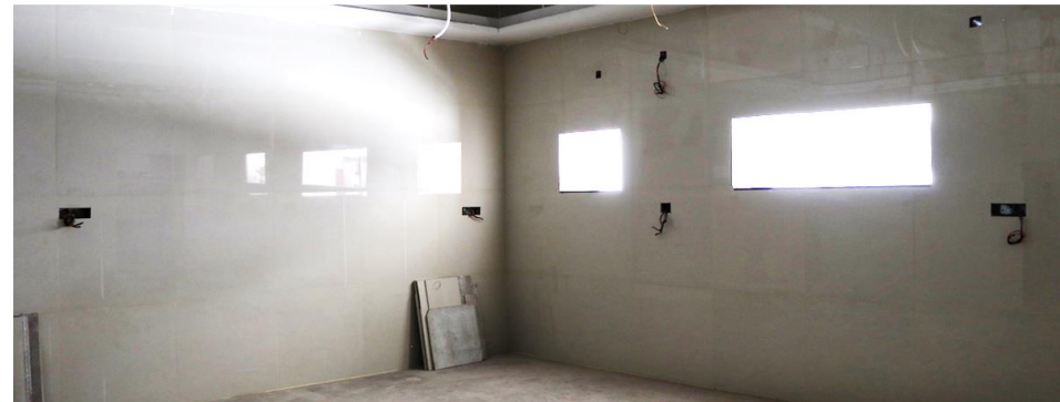
Construction of Multipurpose Hall at Govt. Schools - Madar & Dabok, Rajasthan
