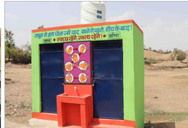
Sanitation facility renovated
